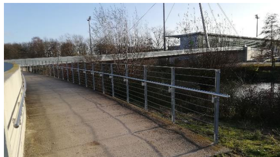
Wheelchair ramp (north)
