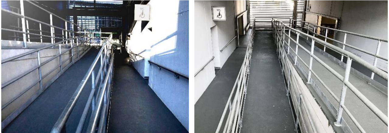
Wheelchair ramp Volkswagen Arena
