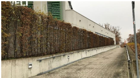
Wheelchair ramp (south)
